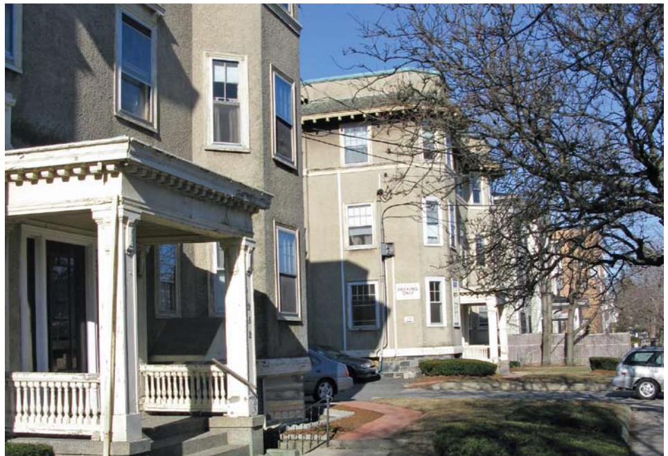
Significant renovations will be made to all 32 apartments, common areas, and exteriors.
